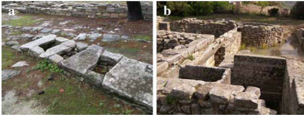
Figure 1. Images of relics of the water system in Tylissos, in ancient Crete. (a) Aqueduct to transport water from springs. (b) Sedimentation deposit (in foreground) with stone channel connecting to cistern (photos copyright by L.W. Mays).
